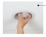
1. Remove the bulb from existing housing.
